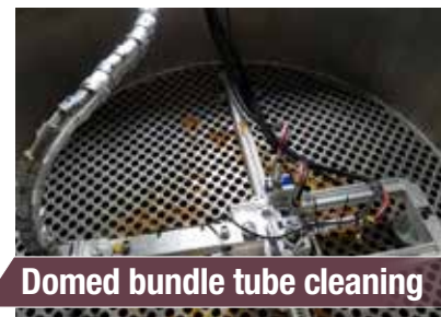
Condenser tube cleaning
