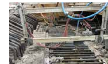
COKE AND REFRACTORY REMOVAL
